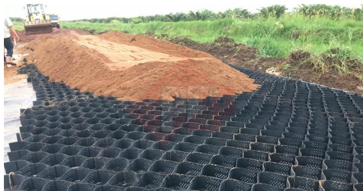
Gambar 5. Pengisian kantong geocell
